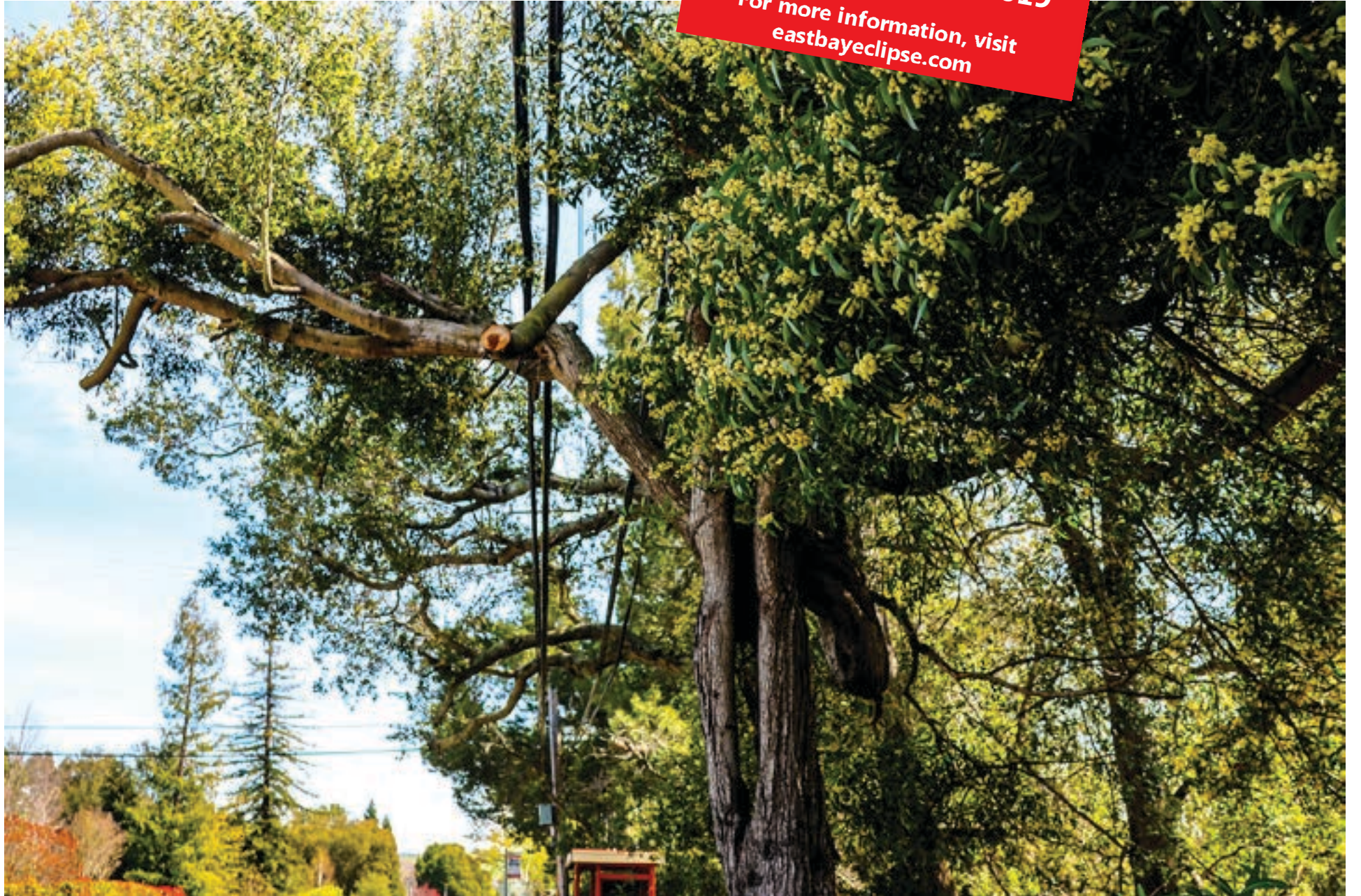
This huge Acacia tree on Moraga Way has been trimmed, but still interferes with wires above it. The trunk is split and the tree is in poor health. Photo Sora O'Doherty
